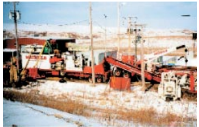
Drilling under permafrost
