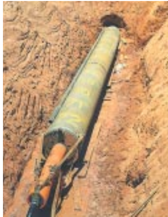
A pipe ramming operation
