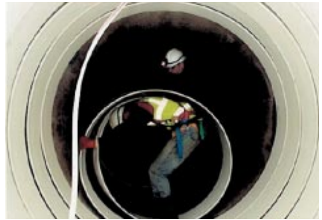
Installing Spiral Wound Lining
