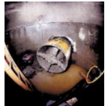
Arrival of a microtunneling TBM at a reception shaft
