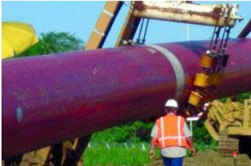
*The Cross Island Pipeline Project in Trinidad involved three HDD bores in the 48-mile installation. The bores were all over 2,000 ft in length and each involved installing 56-in. pipe.*
