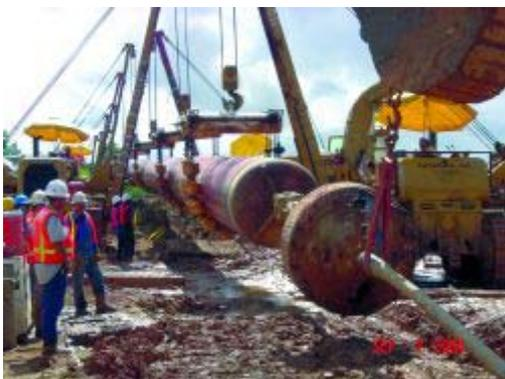
*Each of the three bores required seven reaming passes to reach the 72-in. diameter needed to pull the 56-in. pipe. Due to the size, Southeast Directional Drilling custom-built the reamers for this job.*
